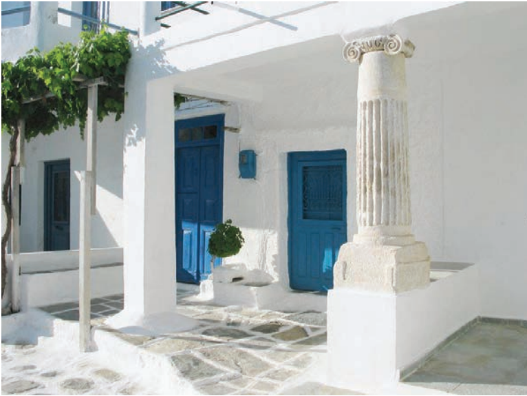
Figure 17. Ionic Column Incorporated to the Local Architecture of a House on the Kastro of Siphnos. Photo Erica Angliker
